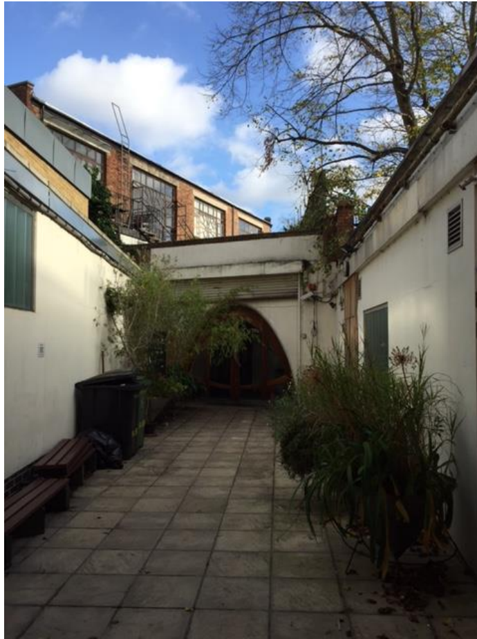
View into the site from the entrance
